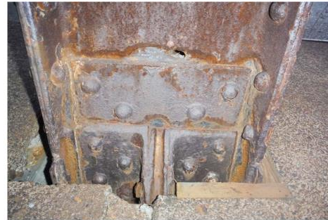
Span 2, Truss B2S – L28U28
