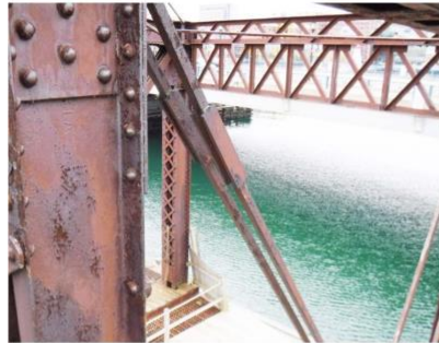
Truss A1N – U9L10 near U9
