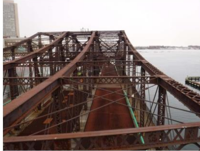
South Bay – West End Bracing (at U9)
