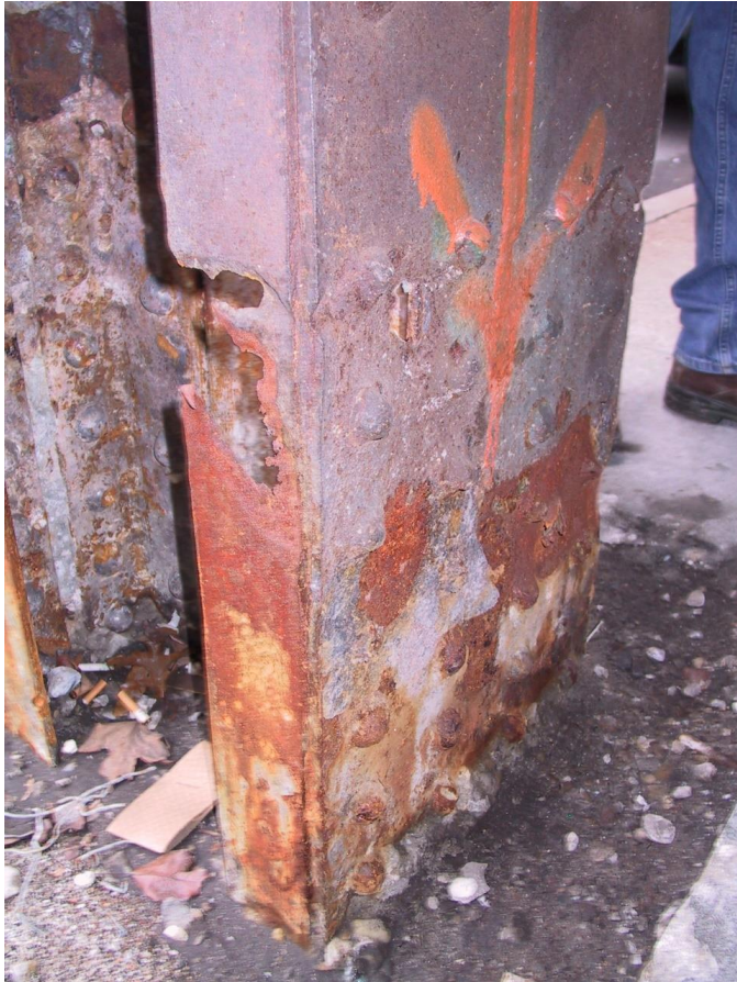
Example of historic steel column repair (non-bridge structure) The High Line (New York, NY)
