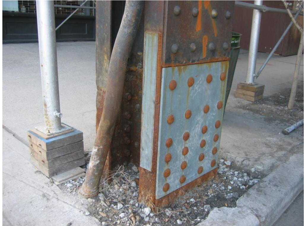
Example of historic steel column repair (non-bridge structure) The High Line (New York, NY)
