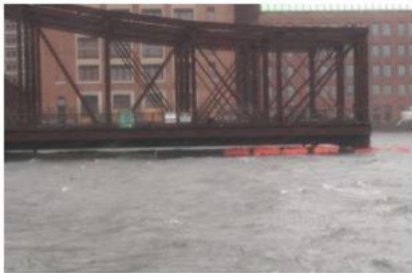
Storm Surge has already brought the harbor to the bottom of the bridge deck.
