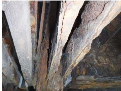
Span 1, Truss A2N – L4L5 at L4
