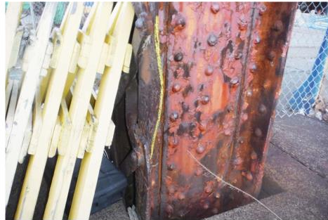
Span 2, Truss B2S - L30U30
