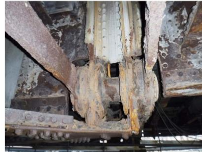
Span 2, Truss B2N – L24L25 at L24
