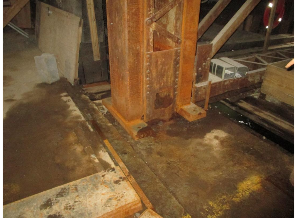
Example of historic steel column repair (non-bridge structure) Battery Maritime Building (New York, NY)
