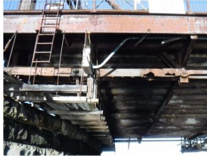
Span 2, Truss A2S – L23L24
