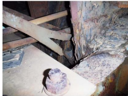
Truss B1N – L16M15 at L16
