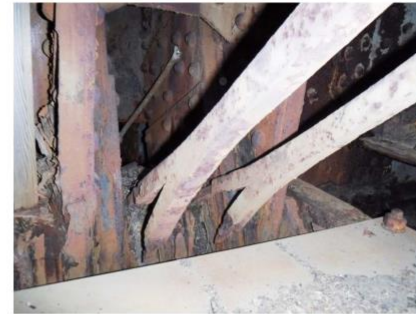
Truss B1N – L15M16 at L15
