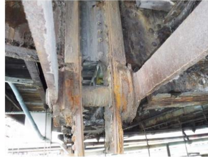
Span 2, Truss A2S – L24L25 at L24
