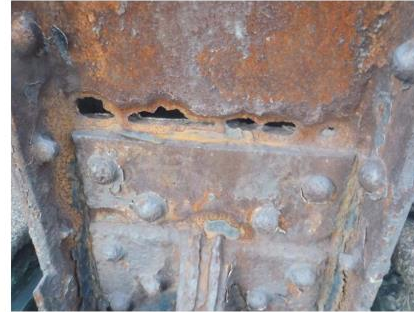
Span 2, Truss B2N – L27U27
