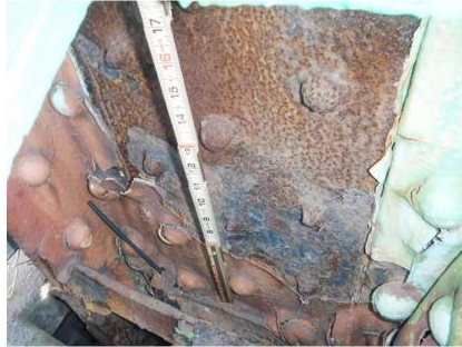
Span 1, Truss A2N – L1U1
